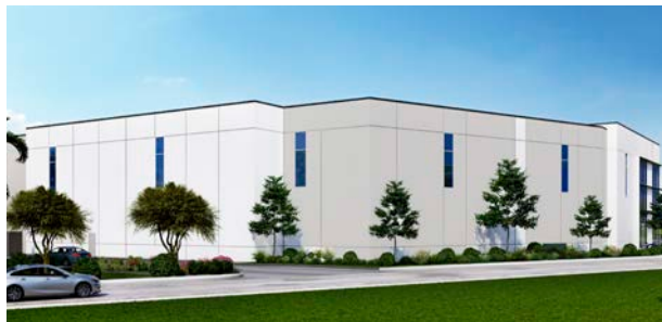
NORTHEAST CORNER STREET VIEW
